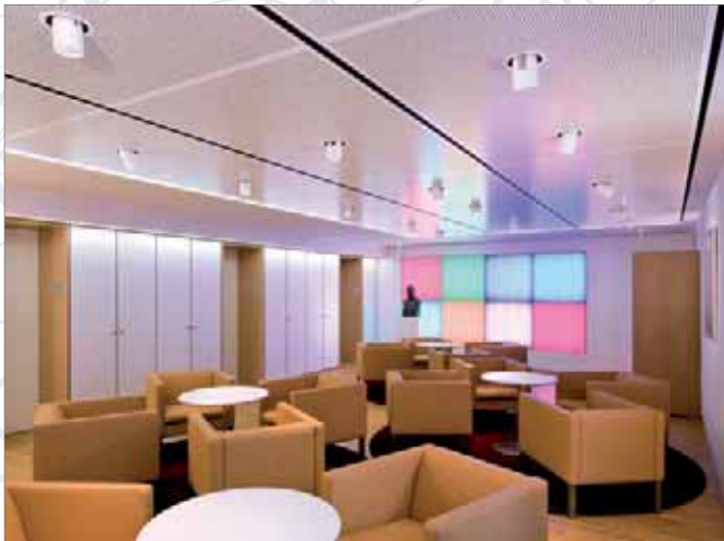
Large modular ceiling with downlights (Munich)
