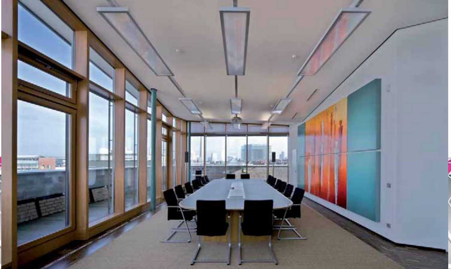
Jointless acoustic ceiling (Düsseldorf)
