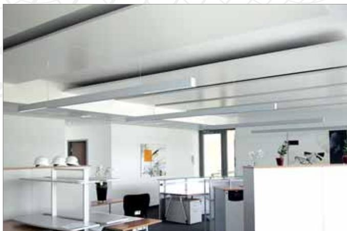
Ceiling sails divided longitudinally with a 120° tilt (Munich)
